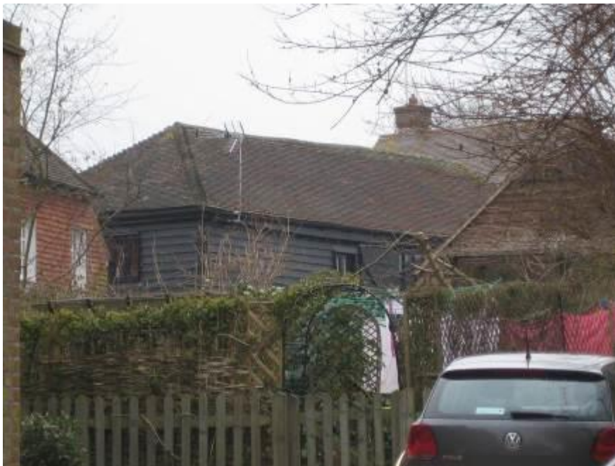
Barn conversion behind Westerham Hall
