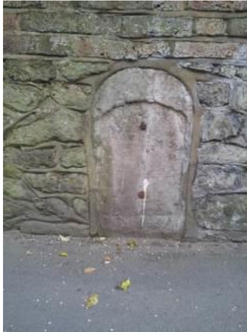
Mile post marker, High Street
